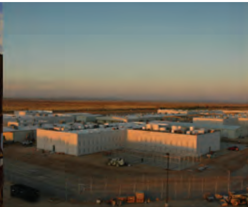
Low Voltage Systems
